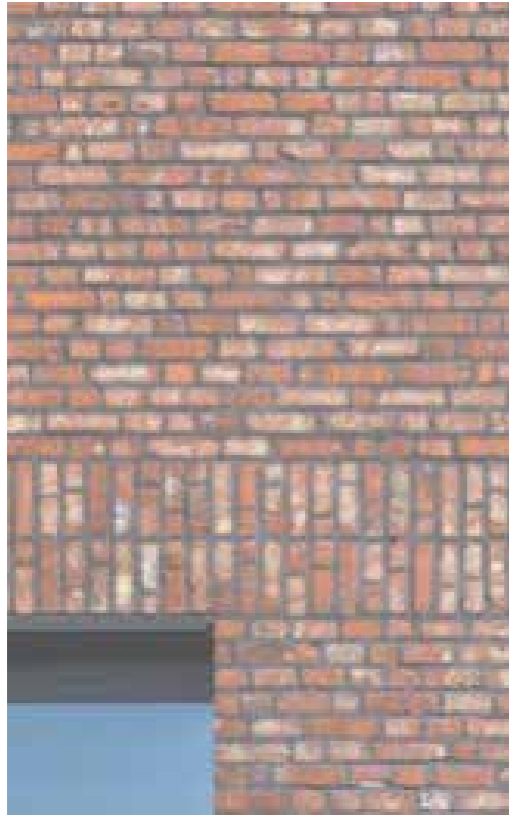
Figure 5.5 - Simple double soldier course detail
