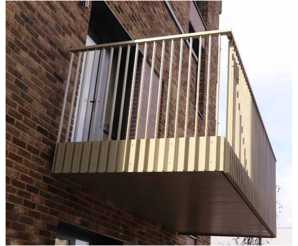
Figure 5.7 - Powder coated vertical steel balcony guarding. Colour can add warmth and distinctiveness.
