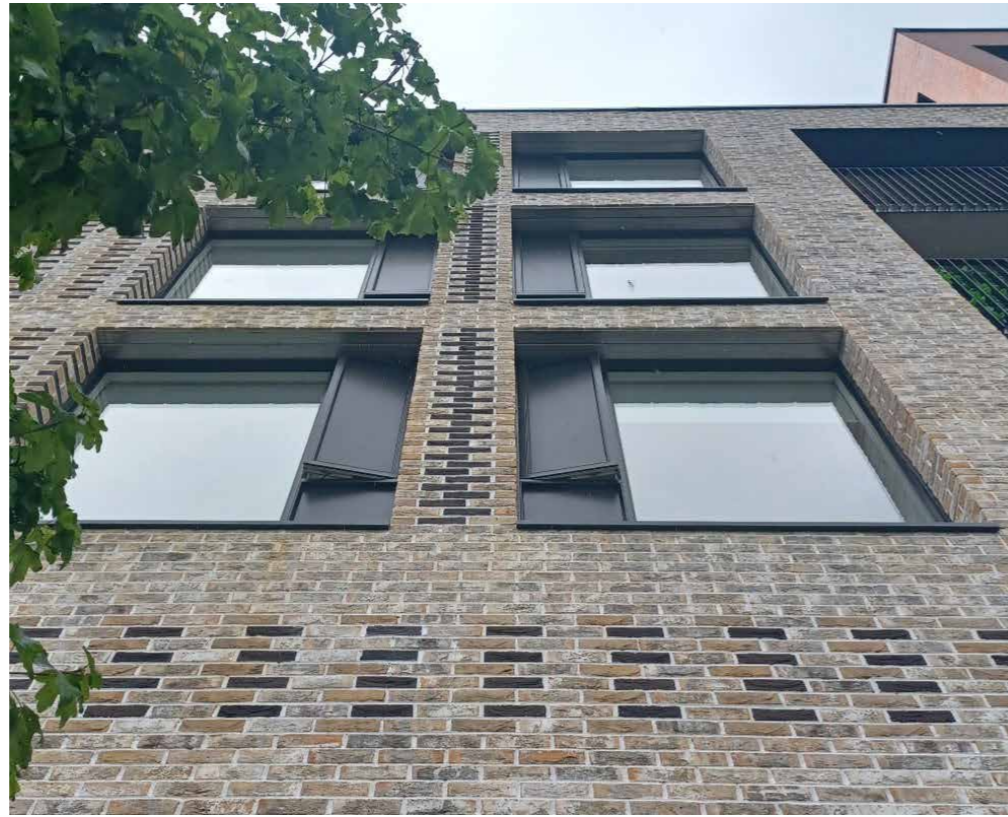
Figure 5.6 - Brick shadow effect similar to recess using dark and buff bricks in the same plane
